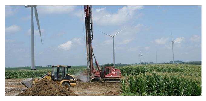
Together, the Rolling Hills Wind Farm in Massena, Iowa and the nearby Laurel Wind Farm provide more than 550 megawatts of power and are some the largest single-phase wind farms in the U.S. Subsurface Constructors installed 7,800 vibro stone columns across a massive, sprawling area to deliver a maximum bearing pressure of 2,500 pounds per square foot. The site consists of loess underlain by deep glacial till with a depth range of 5 to 30 feet
