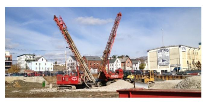
The Bay House provides premium housing in downtown Portland, Maine and required extensive ground improvement work prior to construction. Subsurface Constructors installed 271 <u>aggregate piers</u> to provide a maximum bearing pressure of 3,000 pounds per square foot. The soil profile consists of silt and lean clay (ML) to an average depth range of 3 to 24 feet and sandy soils to an average depth range of about 21 to 34 feet.
