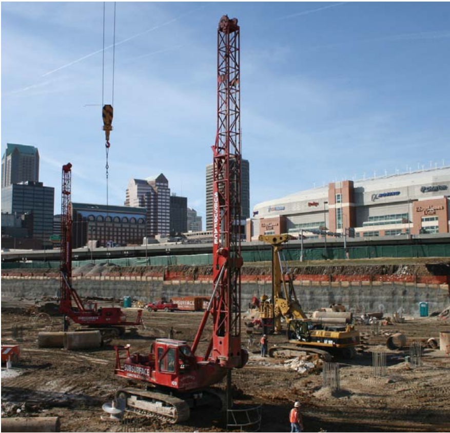
Subsurface was one of the earliest companies in the region to use drilled caissons, a method it continues to use today. Here, work on Pinnacle Casino.
