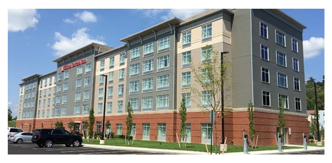
Subsurface Constructors installed 1,005 <u>vibro stone columns</u> to improve the maximum bearing pressure beneath the Hilton Garden Inn of East Boston, Massachusetts to 4,000 pounds per square foot. The soil profile beneath the site consists of 13 to 20 feet of miscellaneous urban fill overlying a two-to-seven foot layer of organic sand on a stiff, silty clay. The site required a 5-foot grade raise.
