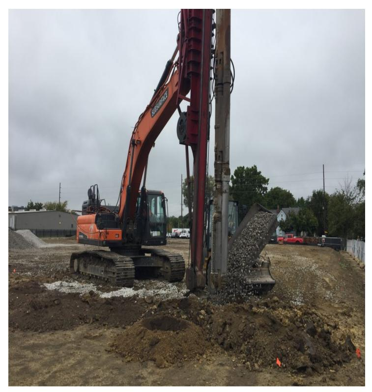
When the soils were just too soft to support the footings for a new YMCA in downtown Springfield, Illinois, Subsurface Constructors helped develop a solution to provide higher bearing pressure using aggregate piers. This
